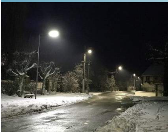
Eclairage public led au Fays
